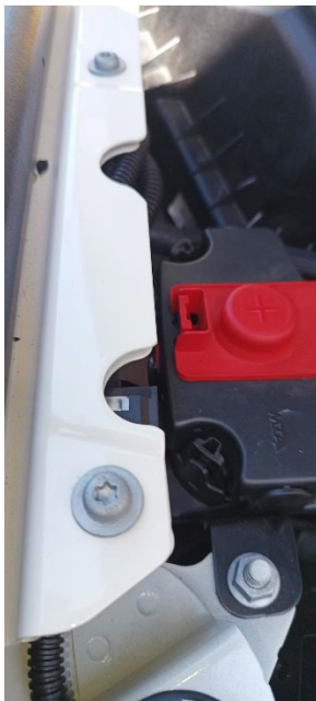
Photo 11: View from above with the relay, wires and connections hidden under the white engine bay lip and secured in place with zip ties.
